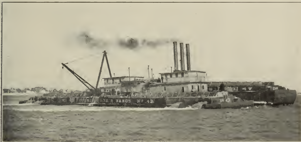
FIG. 30. HYDRAULIC DREDGE NO. 2, NEW YORK HARBOUR, LOADING TWO 1,800 YARD BARGES SIMULTANEOUSLY.
